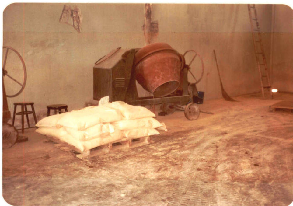
Figure 5.7 A Dry-Mixing Operation for Pesticides, the Floor Area is not Clean
