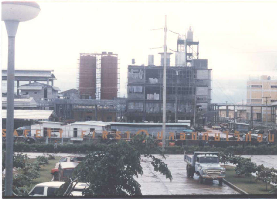
Photo_7 A Petrochemical Plant in Operation, Rayong
